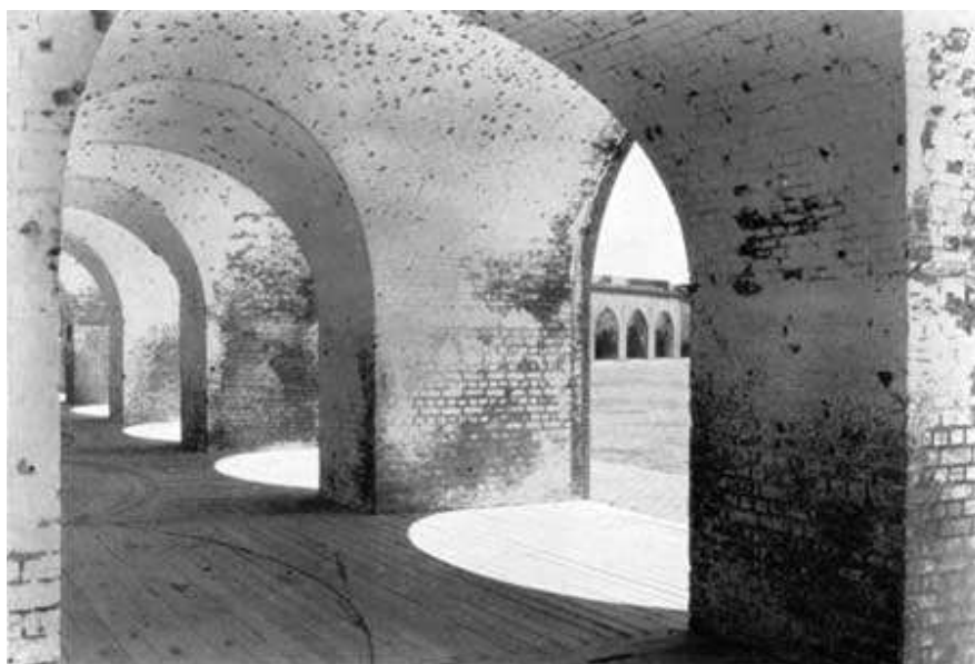
A view from the great brick archways of the casemates into the parade.
