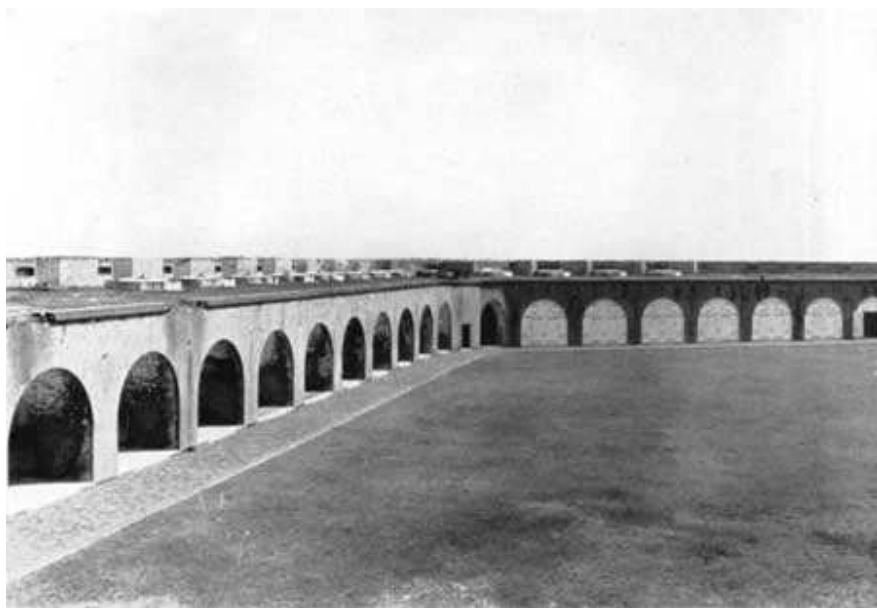
Looking across one corner of the parade toward a section of open casemates and a contrasting tier in which the wooden casemate fronts have been reconstructed.
