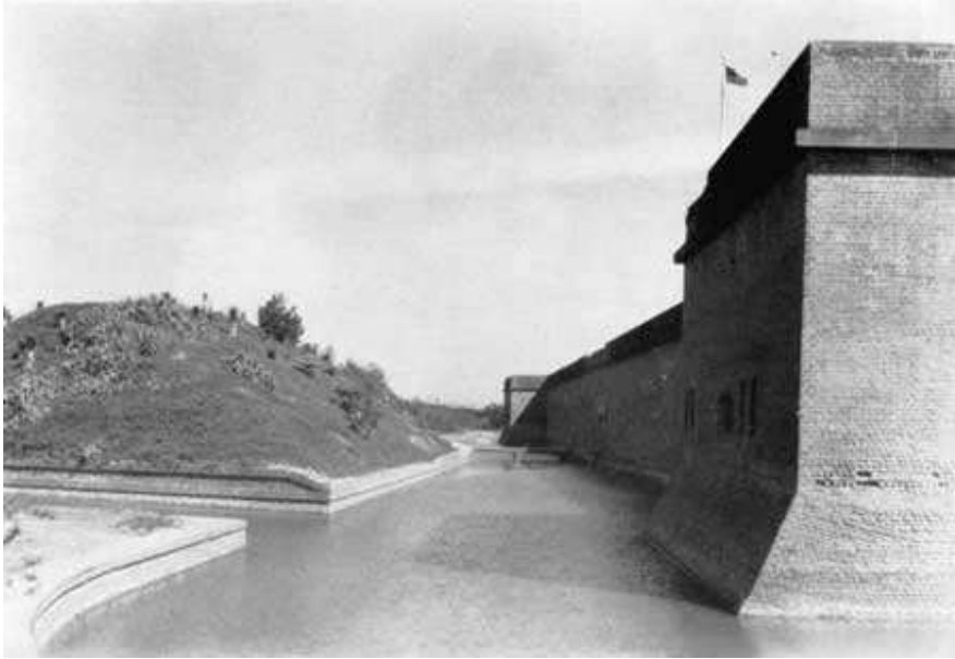
Rear wall of the fort, showing the moat, bastions, drawbridges, and sole entrance through the sally port.
